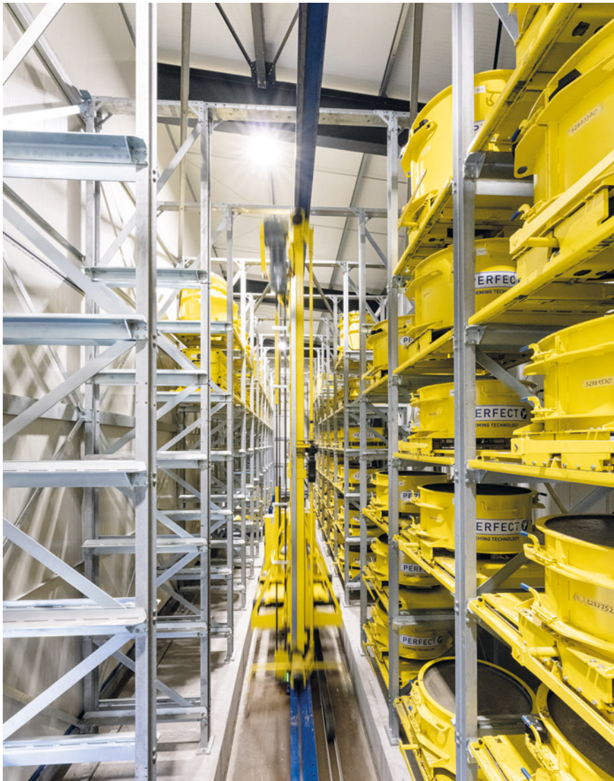
In order to make optimum use of industrial halls, rack systems are ever more frequently being used alongside cranes to provide dedicated hardening zones.
