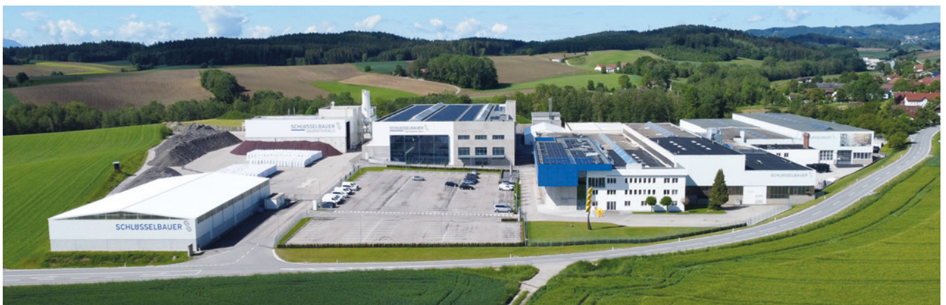
The Schlüsselbauer headquarters in Gaspoltshofen
